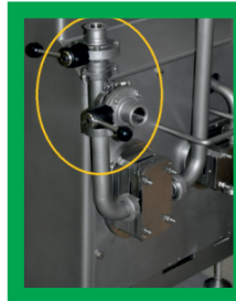
manually operated by-pass valve
